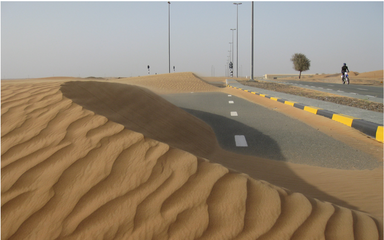
Dunes migrate across a newly built road (Photo credit: David Thomas).
